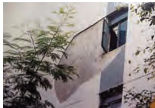
Concrete buildings in Hong Kong, though impressive, suffer from the same problems experienced by concrete the world over. That is, they contain steel reinforcement, which readily rusts in the humid atmosphere that prevails here through most of the year. In addition, the surfaces of many buildings are rendered over and some are also tiled. Joints to allow for movement are seldom incorporated in the surface and as a consequence often pieces fall off. Maybe they should be fibre reinforced!
